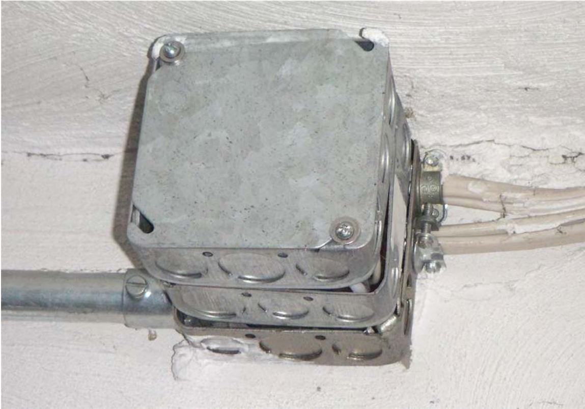
Figure 18. Stacking two additional square junction boxes atop an existing one created room to install common-mode chokes on the four Romex-cables seen at right. Each choke was a 5943003801 toroid wound with three insulated AWG 12 or 14 wires (matching the wire gauges of the respective Romex cables). Connections were made with standard wire nuts.
