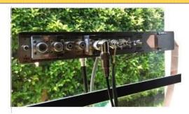
This worked out very well and I now have a quick disconnect capability with feed-throughs and a bulkhead plate for grounding the shack. The up side is I can disconnect the station from the outside world in 20 seconds. Great for when those pesky thunder storms pop up in the summer time.
