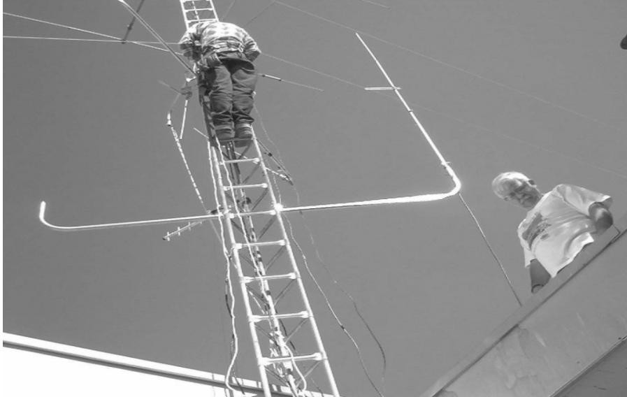
Freddie KF4FCW scales SPARC clubhouse tower to install new VHF-UHF antennas as Dee N4GD checks the installation.
