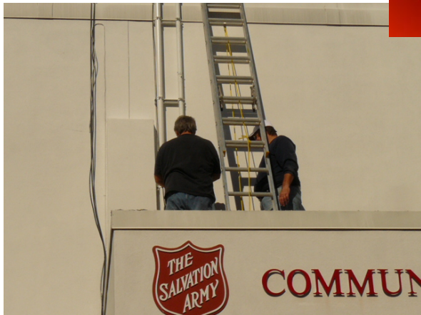
John, KI4UIP, and Bob, N2ESP, installing the center mast.
